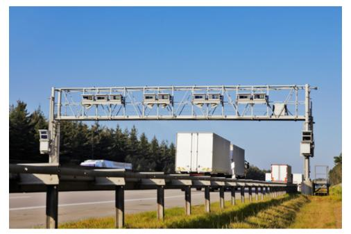
Lidar can significantly increase the accuracy of gantry-based electronic tolling systems, which have been widely deployed in the U.S. to enable free-flow toll collection.
